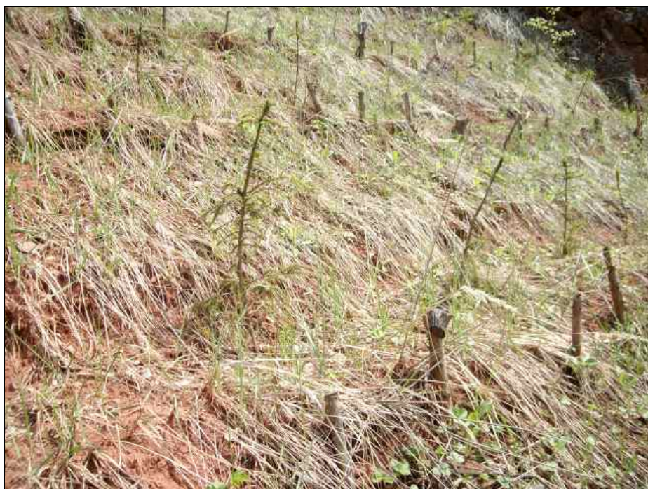
Fig. 4 Aspect with erosion on the hillside with slope of 10 % with mattresses and with spur – tree planted
