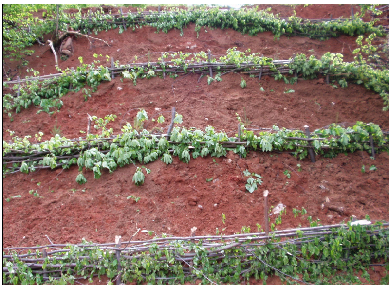
Figure. 1. Beech tree mattress after being set up (2004), in the former bauxite quarry from Zece Hotare, Bihor
