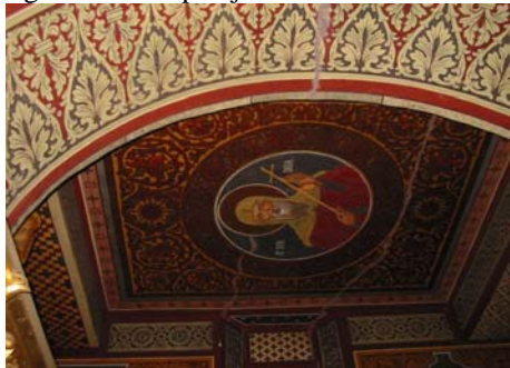
Fig.3. Cracks at arches and vaults
