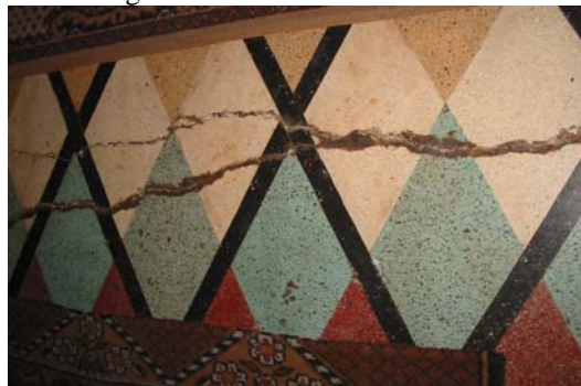
Fig.4. Cracks in the floor
