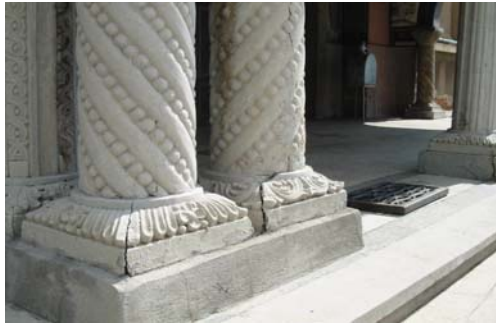
Fig.2. Cracks/open joint fissures at columns
