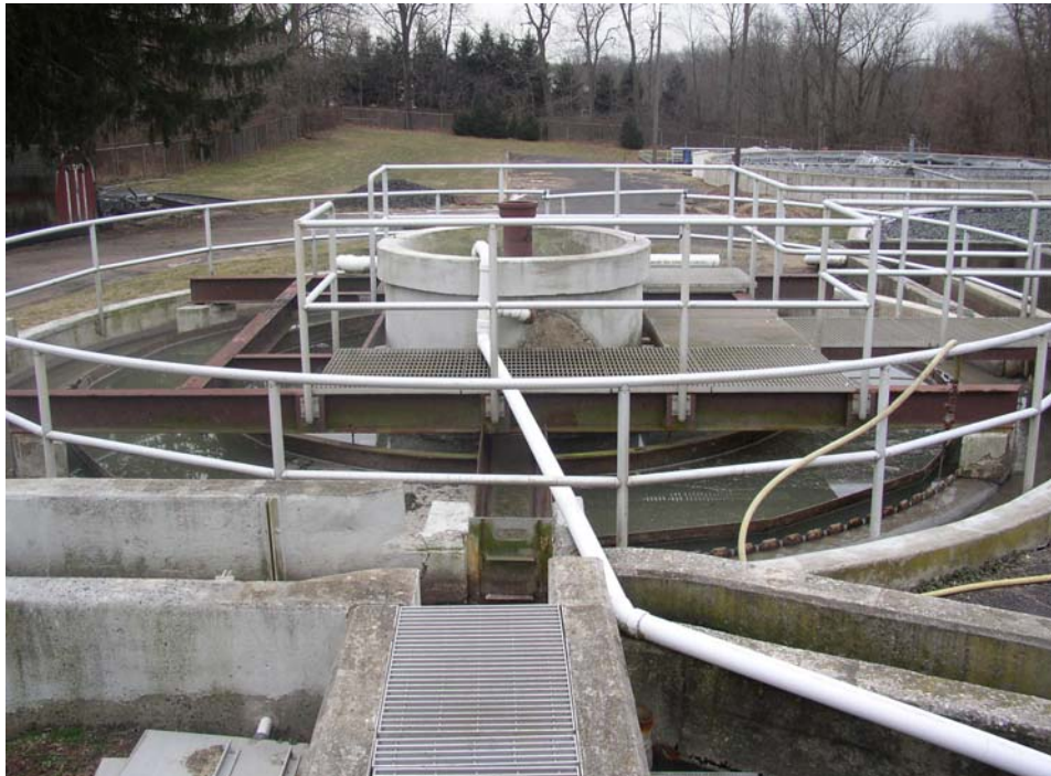
Fig. 1. An original circular Imhoff tank constructed in 1914 ( www.keystone-alliance.com/.../P1190008.jpg )
