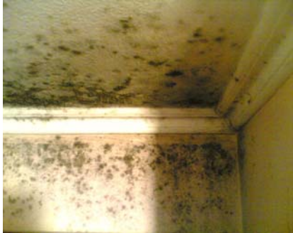
Fig. 2. Mold/dampness to unheated superior apartment
