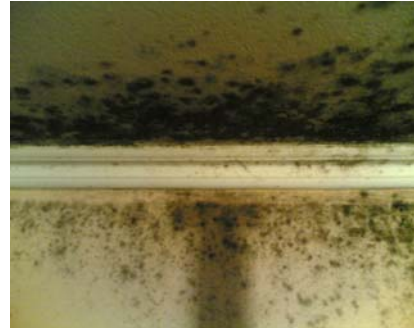
Fig. 3. Mold/dampness unheated upper floor
