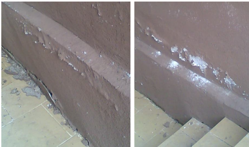
Fig.5 Case study, carbonation phenomenon at the retaining walls
