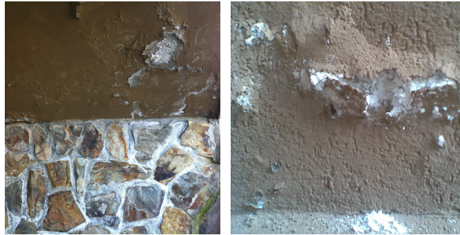
Fig. 4 Carbonation phenomenon
