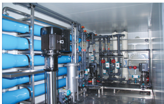
Figure 1 System of water treatment in a container
