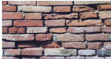
Fig. 1. The action of the ascending water in a historic masonry with cement mortar
