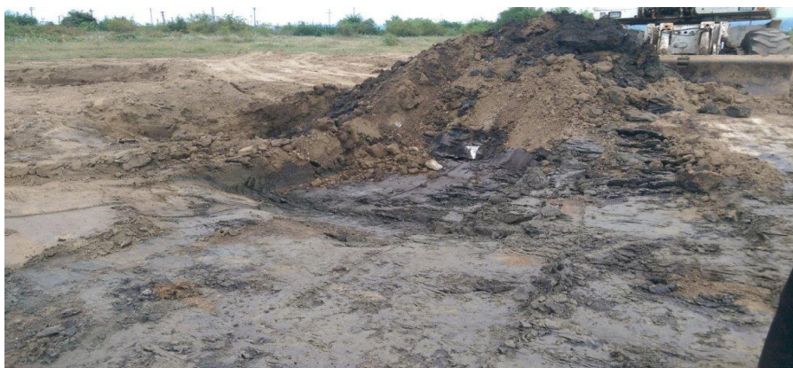
Fig. 2. The excavation of the soil contaminated with petroleum residue from the perimeter of the Suplacul de Barcau locality
