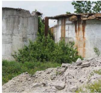
Fig. 3. The area of chemical preparation (fire pumps, water tanks, electric station)
